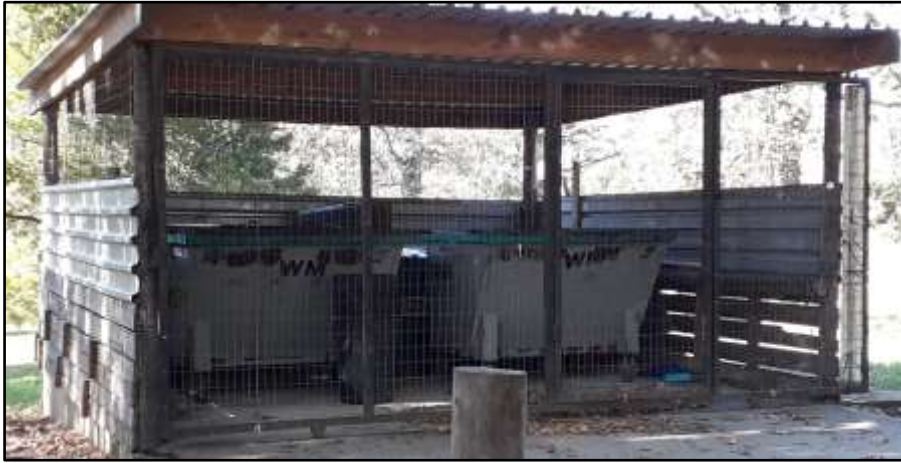
Figure 10: Secured and clean waste cage at Chrysalis Academy on 4 May 2020.
